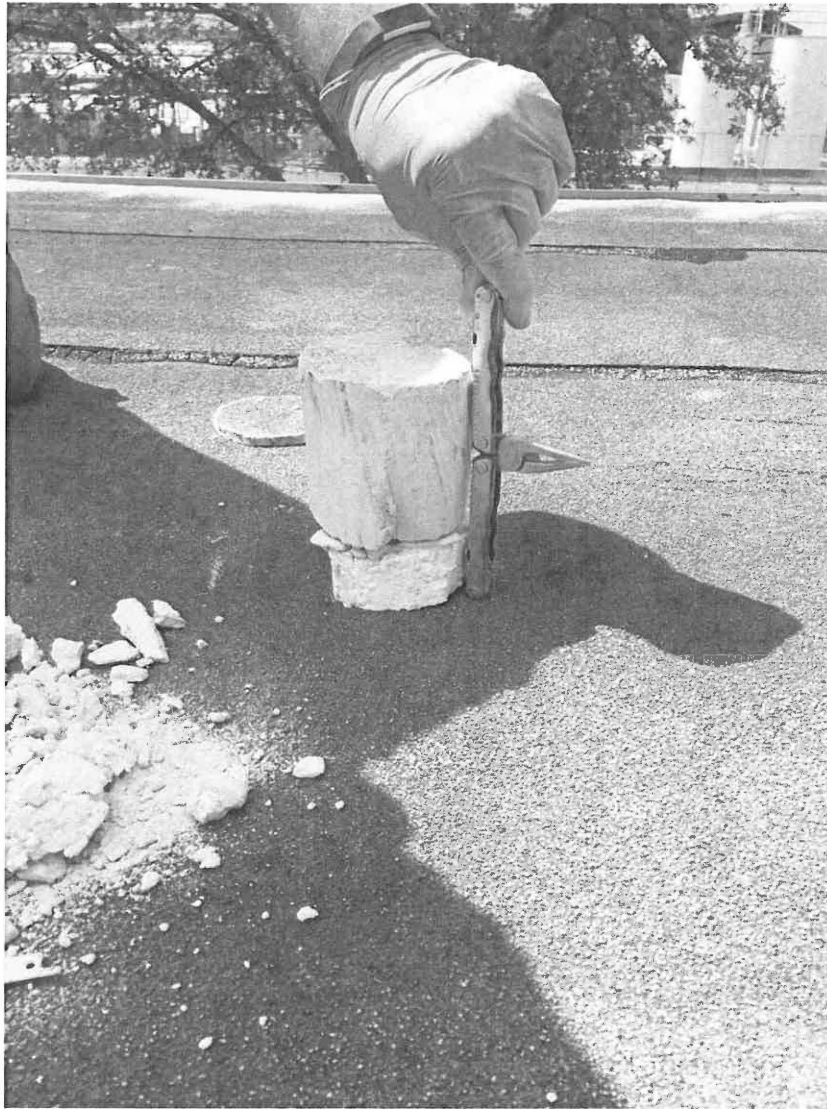
Photo 2: 6" core (2" foam and 4" fire clay) Original roof center of building. Core from Southwest side. 10,920 sq feet.
